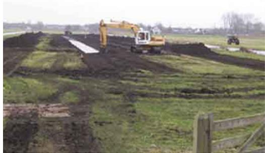
Figure 6. Creation of a new ditch in the Uithoorn Polder (Noord-Holland) (Photo: H.H. de Vries).
